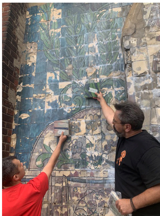
Fig. 16 a, b. Selection of the color of the glaze for the western portal. On the left is the head of the restoration work, K. V. Likholat. Photo "Pallada", 2023
